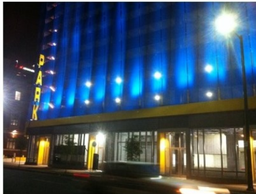
*ACTUAL PICTURE OF PARKING GARAGE*
